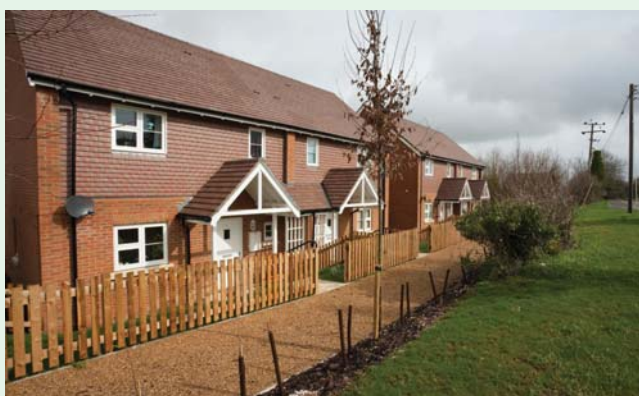
Streetway Road, Grateley
