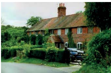
Typical terraced farmworkers' cottages, Tunworth
